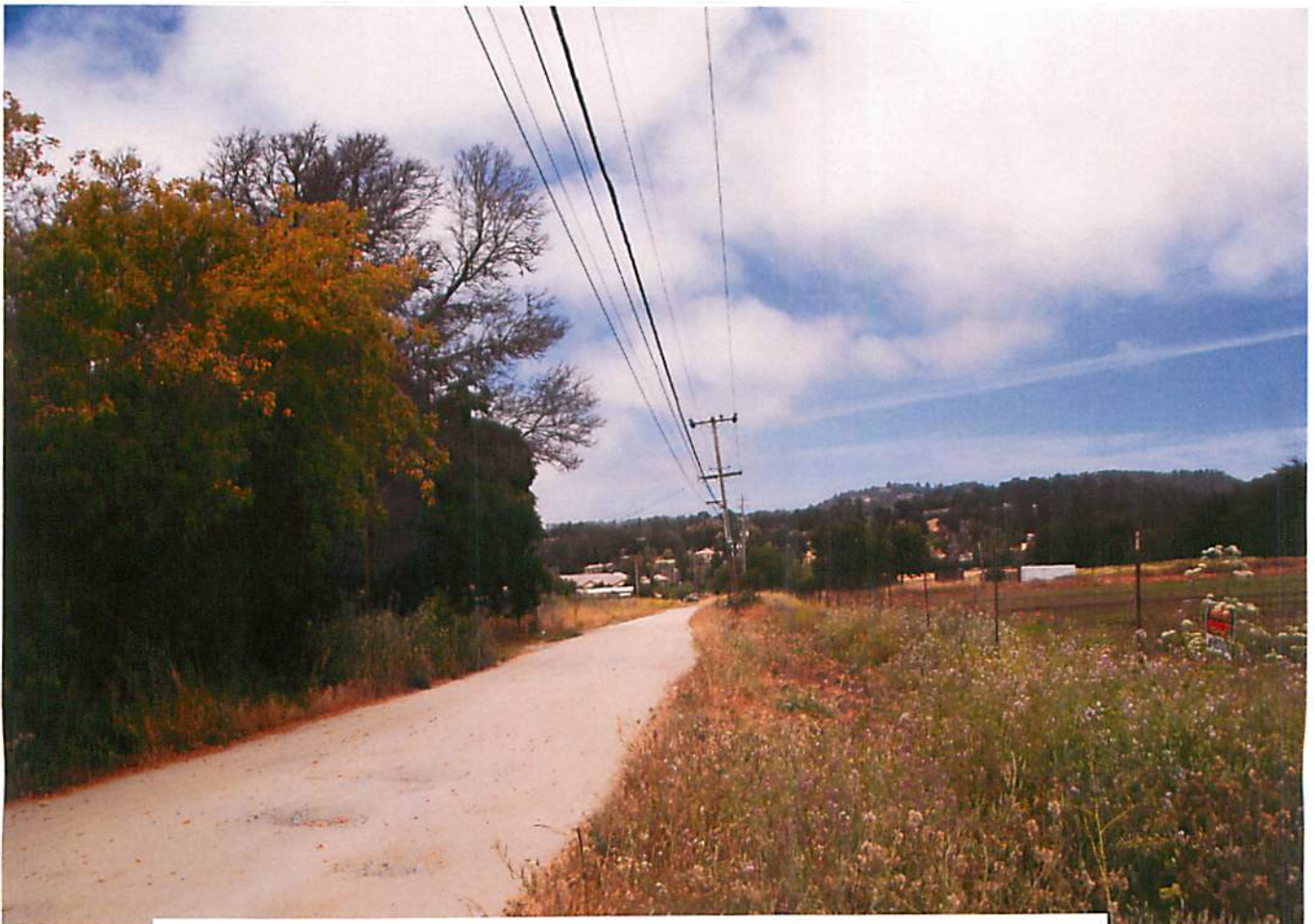
#2 Val Verde Drive - Private Road Existing Conditions View: South to North
