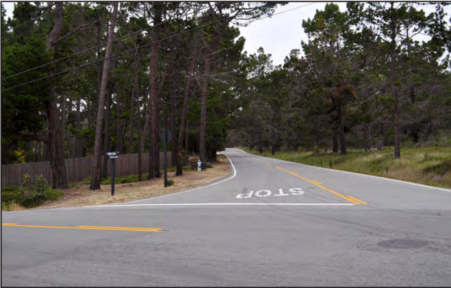
20. Looking northwest from the Ronda/Viscaino Road intersection toward Area I-2.
