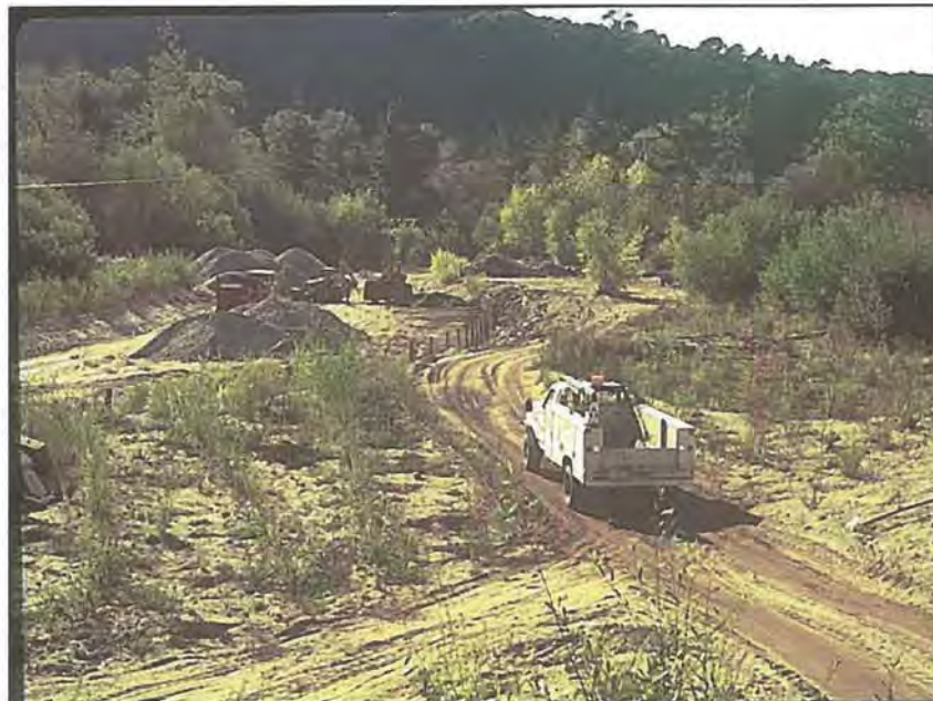
November 1993 – Installing the channel grade control structure and post/wire revetment.
